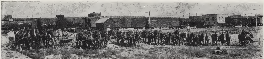
The Willis Construction Crew. Photograph taken at Grey Bull, Wyoming, just after the railroad was built in 1914.
