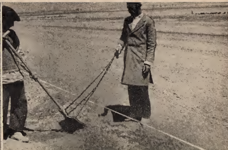
Men making a dike for irrigation. One shovels and the other pulls on a chain attached to the shovel.
